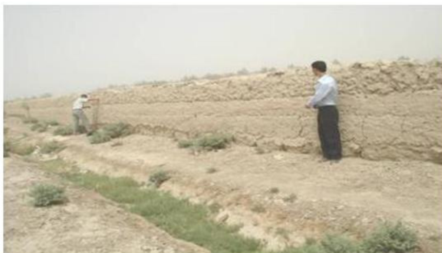
Figure 2. View of Mud wall wind break which used in this study as an abiotic windbreak
