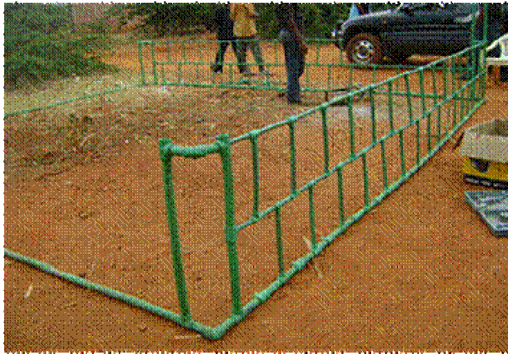
Figure 5. An incomplete cage undergoing fabrication.
